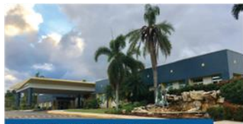
Metro Pavia Clinic Arcibo
